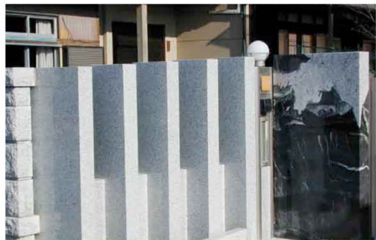
03 門(袖石、稲田みかげ) 150mm × 900mm × 1500mm × 1 150mm × 400mm × 1500 ~ 1650mm × 4 150mm × 600mm × 1700mm × 1 150mm × 200mm × 750mm × 4
